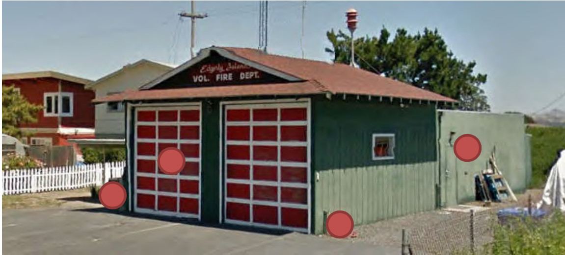
Figure 3 Summary of potential structural deficiencies at the existing fire station.
